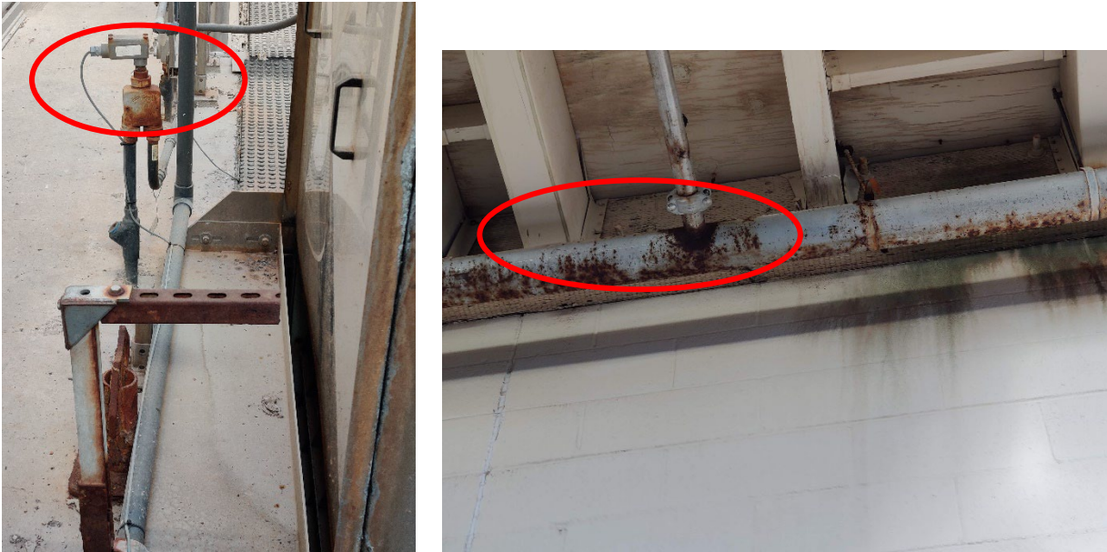
Figure 6-14. Typical H 2 S Corrosion of the Electrical System and Fire Sprinklers
