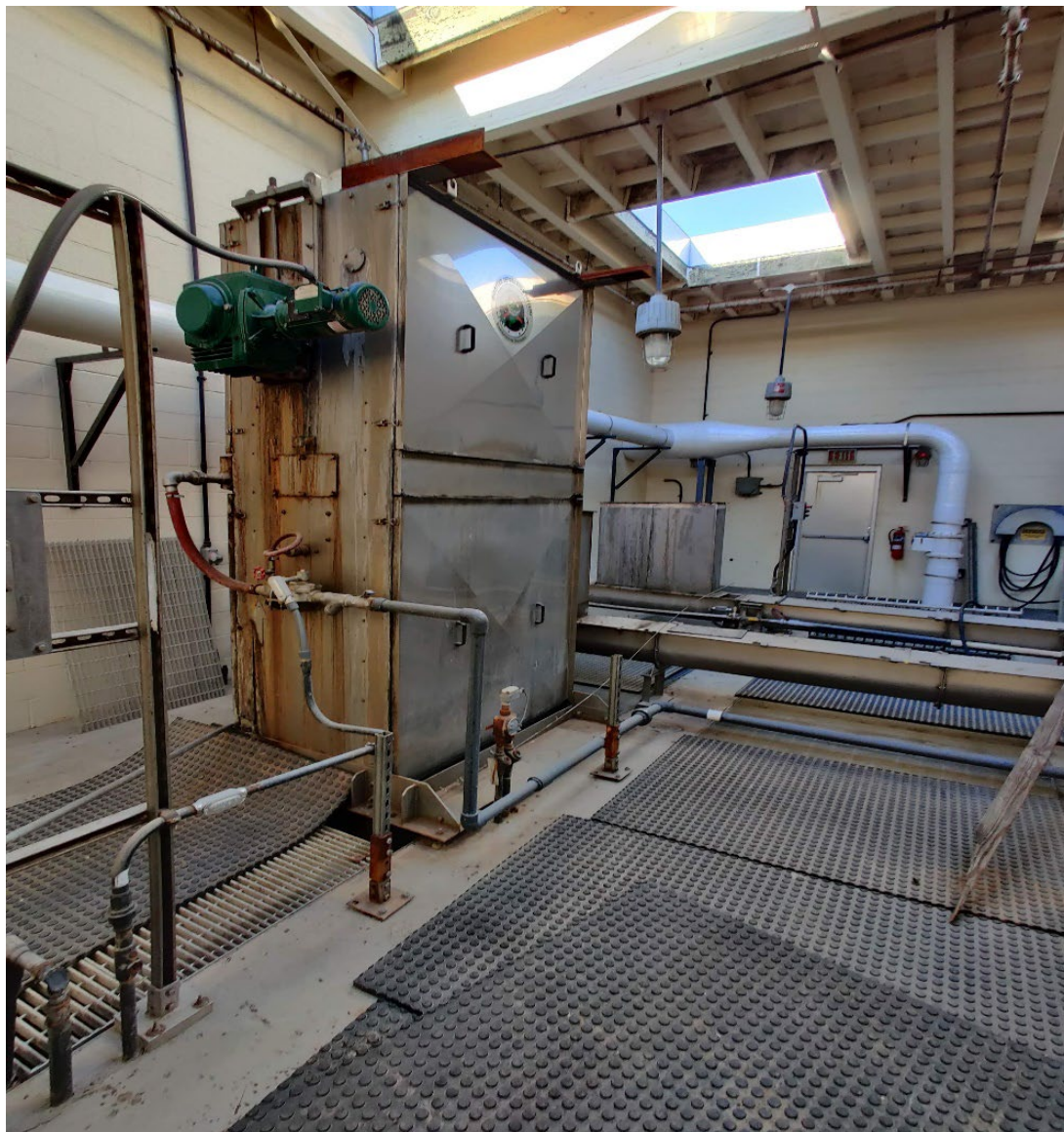
Figure 6-13. Screen Enclosure Showing Signs of Corrosion
