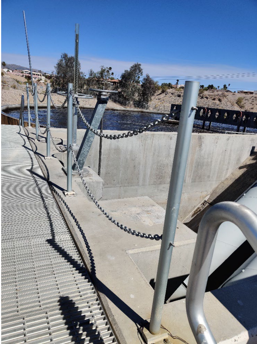
Figure D-9. Chain Railing Installed at the Top of the RAS Sump Pit; RAS Pumps are Located to the East
