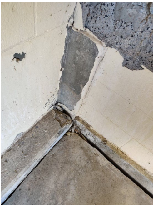
Figure 6-6. Cracks Observed in the South Wall of the Headworks Building
