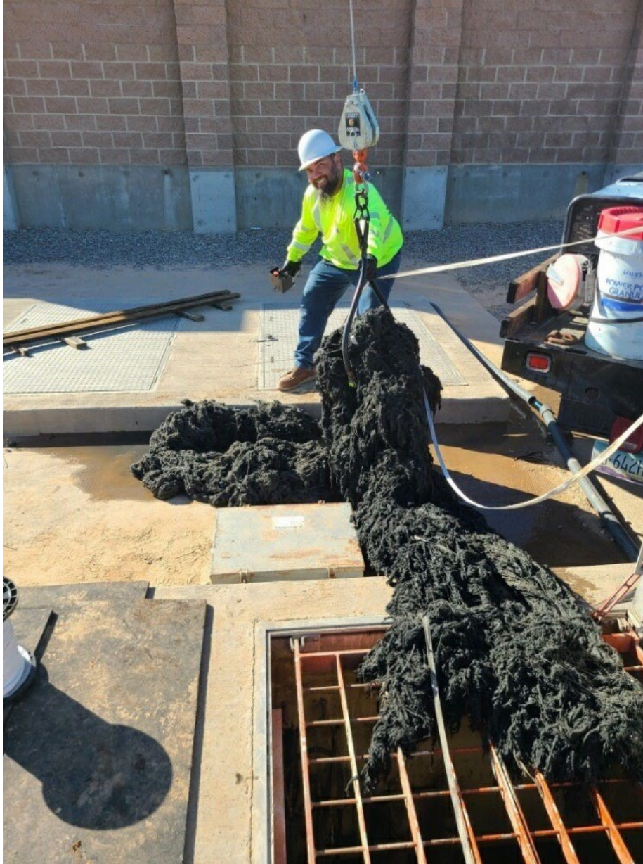
Figure 5-5. Rag Ball Being Removed from the Bombay Pump Station
