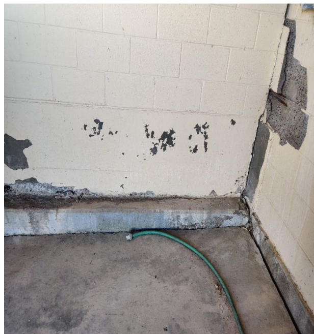
Figure 6-6. Cracks Observed in the South Wall of the Headworks Building
