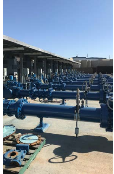
WTP Photos from site visit on 2/22/18
